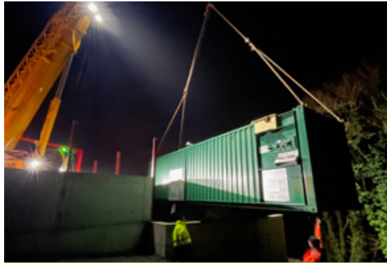
On-site installation : UK, 2025 sawdust drying / 2.800 kg/h
